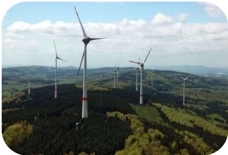
Windpark Soonwald, RLP (70,5 MW)
